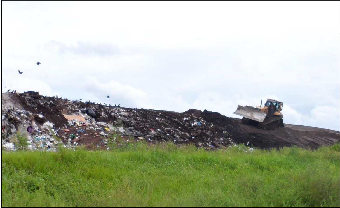
Photo 1. Orange County Landfill
